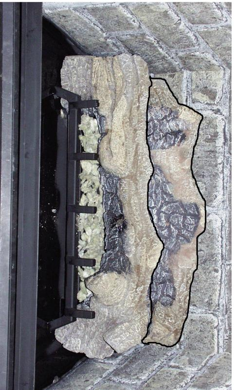
**Step (6)** Place rear log on to the log retainer 1/2" away from back of fireplace. (If refractory liner is used, make sure refractory liner is installed first then back log is to be pushed up against it as tight as possible.)
