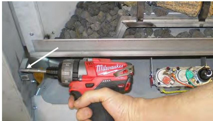
Step 2 (illustrated): Install screws in top corners. Attach left and right Access Panel Brackets to inside of face frame with DT Screws. Lower Face Panel will now be openable.
