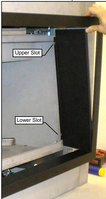
**2.** Attach Side Filler of Surround to firebox face with two screws. Repeat for other side of fireplace.
