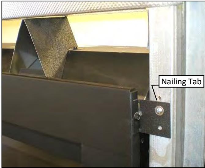
**Step Two:** Use Drywall to finish face of wall. **NOTE:** Drywall will be flush with fireplace face.
