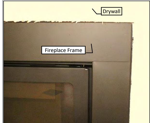
**Step 3:** A stone, brick, or other non-combustible border may be applied to the wall. Maintain clearances from fireplace opening below.
