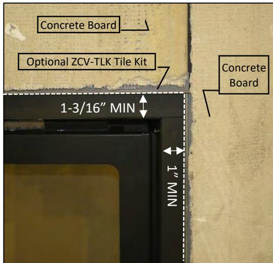
**IMPORTANT NOTE!:** If installing tile, brick, or other non-combustible material around the perimeter of the S2PF2 Surround, Maintain clearances shown below. Also See Basic Finishing 4.
