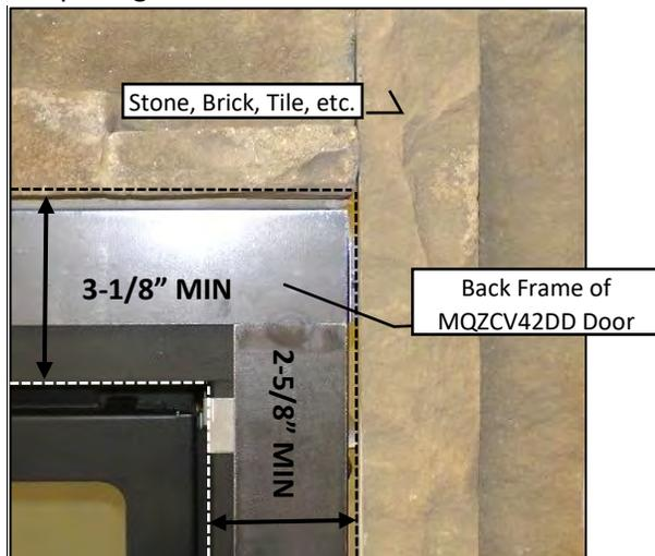
**IMPORTANT NOTE!** When installing stone, brick, or other material around the perimeter of the surround: You MUST Leave 2-5/8" of the fireplace face exposed around the fireplace opening on the Sides, 2" at the Bottom, and 3-1/8" must be exposed on the top. This is to install and remove the Door Frame. See drawings below.
