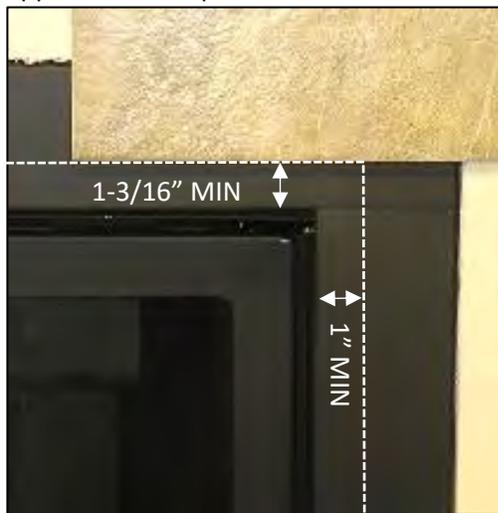
**IMPORTANT NOTE!** If installing tile, brick, or other non-combustible material around the perimeter of the screen: you **MUST** Leave 1" of the face exposed around the fireplace opening on the Bottom and Sides, and 1-3/16" exposed on the top. This is to install and remove the safety screen. See drawings below. **A Tile Lip Kit is Available. Part No. ZCV-TLK**
