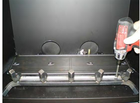
Place Glass Tray over Burner. Insert Pilot Cover into slots in Glass Tray.
