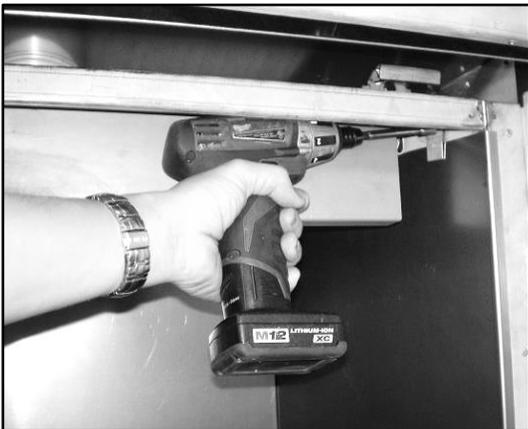
**Step Four:** Fix Side Liners in place using Liner Retainer Clips.
