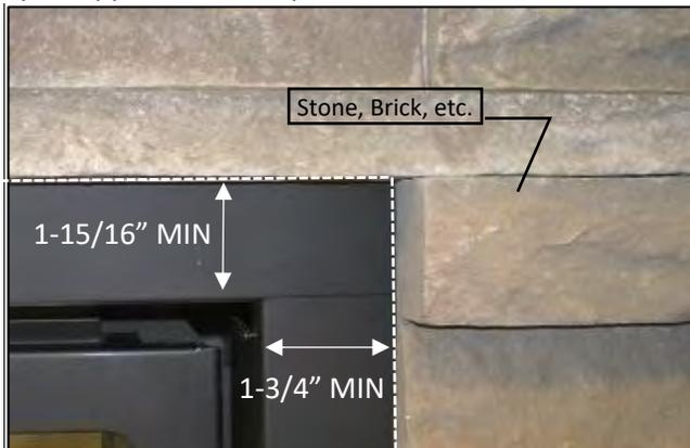
**IMPORTANT NOTE!** If installing stone, brick, or other non-combustible material around the perimeter of the surround: you MUST Leave 1-3/4" of the face exposed around the fireplace opening on the Bottom and Sides, and 1-15/16" exposed on the top. This is to install and remove the surround. See drawings below. **A Tile Lip Kit (ZCV-TLK) is available.**
