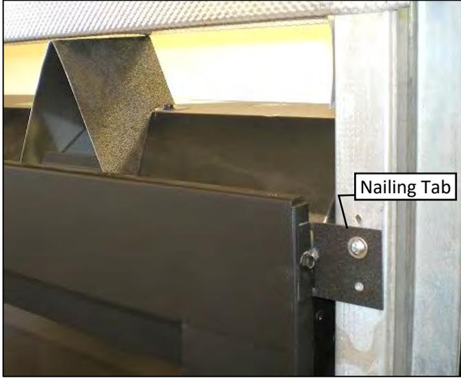
**Step Two:** Use Drywall to finish face of wall.
