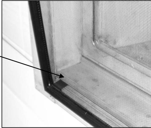
Push top of screen up against fireplace and hook onto screws in side frame. Push down on screen to lock in place.
