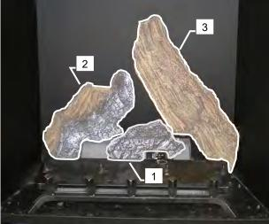
Logs 1-3 are placed against back wall of firebox.
