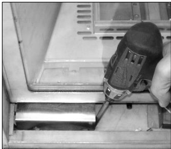
Power Vent Control Module Mounted inside fireplace.
