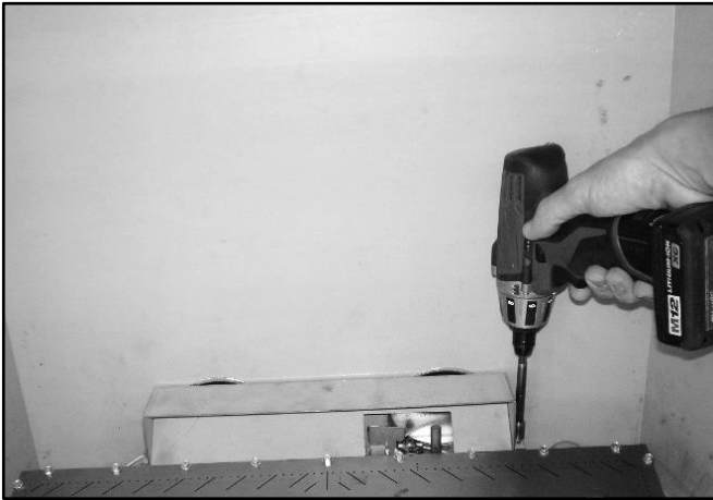
Step One: Remove Log Holder.
