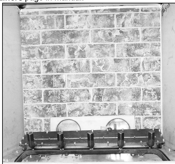
Step Two: Place Back Liner against back wall of firebox.
