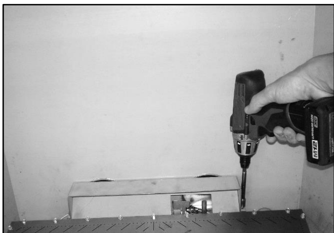
Step One: Remove Log Holder.
