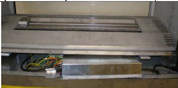
Remove Glass Doors from both sides of fireplace. Remove UHS Box from bottom of fireplace.
