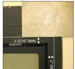
**Step Two:** Use Non-Combustible Header Strip on top frame of fireplace and Drywall to finish face of wall. **NOTE:** Drywall will be flush with fireplace face.
