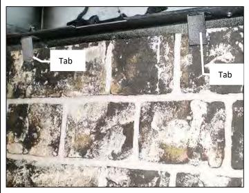
NOTE: Brick Liners MUST BE CUT and installed AFTER MST42GT is installed.
