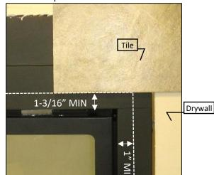
**Step Two:** Use Non-Combustible Header Strip on top frame of fireplace and Drywall to finish face of wall. **NOTE:** Drywall will be flush with fireplace face.
