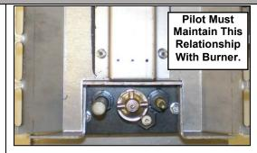
Refer to "Gas Specifications Chart" for inlet pressures and input ratings. Clock meter to verify input rate. Place conversion label as close to converted gas control as possible. Refer to lighting instructions to verify the normal operating sequence of the ignition system.
