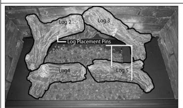
**Step #3** – Place Logs 2-3 on top of Log 1, Locate holes On bottom of logs 4-5 and place these onto Log Placement Pins as shown in the Photograph above.
