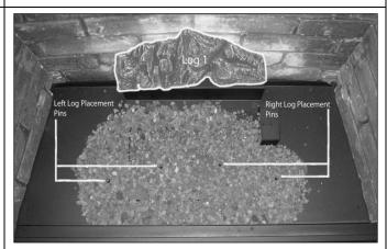
**Step #2** – Place Log 1 onto Rear Log Holder and up to Brick Panel.
