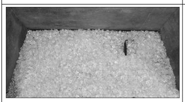
Step #2 - Place Glass onto and around Burner Pan as shown, do not place glass into the Pilot Shield assembly area. NOTE: It is not necessary to place rocks over glass.
