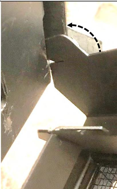
**2: Raise Screen.** Ensure that Lower Hooks remain engaged. Top Hook is directly above Slot.
