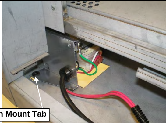
Set fan onto Mount Tabs inside fireplace.
