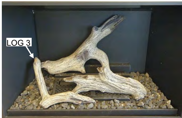
STEP 3: Place LOG 3 on left side of firebox as shown.
