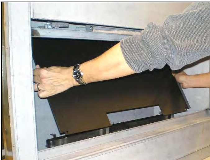
Insert Back Liner. Tilt Side Liners into place and attach to firebox with Screws removed from sides of firebox. Replace all components.
