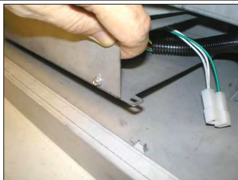
2. Lift UHS Box out of Unit
