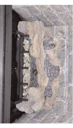
**Step (6)** Place rear log on to the log retainer 1/2" away from back of fireplace. (If refractory liner is used, make sure refractory liner is installed first then back log is to be pushed up against it as tight as possible.)
