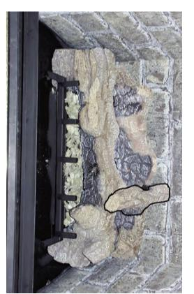
**Step (7)** Place right crossover log across front and back logs using the log placement pin as a guide.
