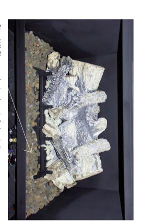
**Step (9)** Position Log (8) up against the 3rd grate post from the right, and position upper section of Log (8) against Logs (2) and (7). **Step (10)** Place crushed rocks onto firebox bottom. (NOTE: Do not place crushed rock onto burner tubes)
